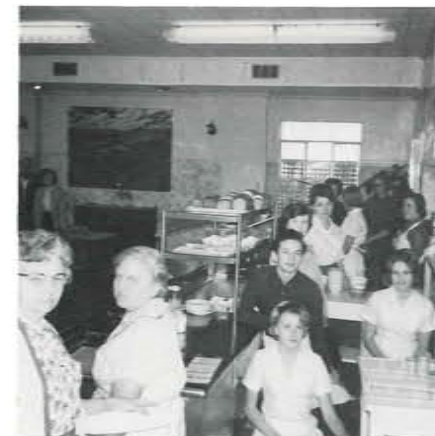
CAFETERIA HOSPITAL KITCHEN
