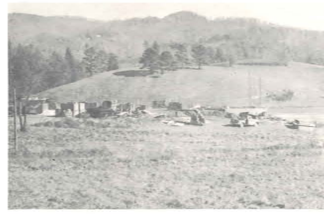
Construction "Boy's Dorm"
