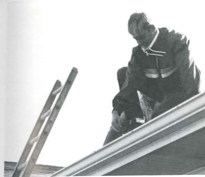
Todd Mace carefully cleans out the gutters.
